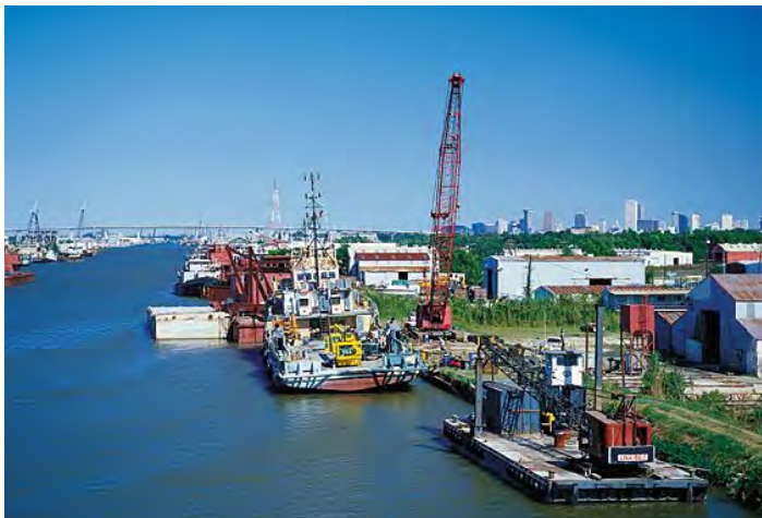
Improvements of the levees along the Harvey Canal are necessary for the long-term protection of the Terrytown study area from storm surges from the south. 3
