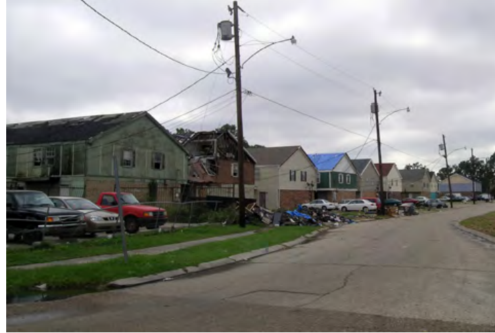
Damaged and vacant buildings interspersed with habitable ones create a blighted, unsafe streetscape along Nell. Garbage has piled up and cars block the sidewalks.
