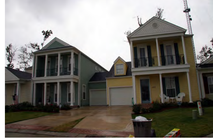
These are the Plantation Townhomes being built in the new Hamilton Oaks subdivision. The wide balconies create shaded outdoor living space, an important climate-sensitive design in this hot region.
