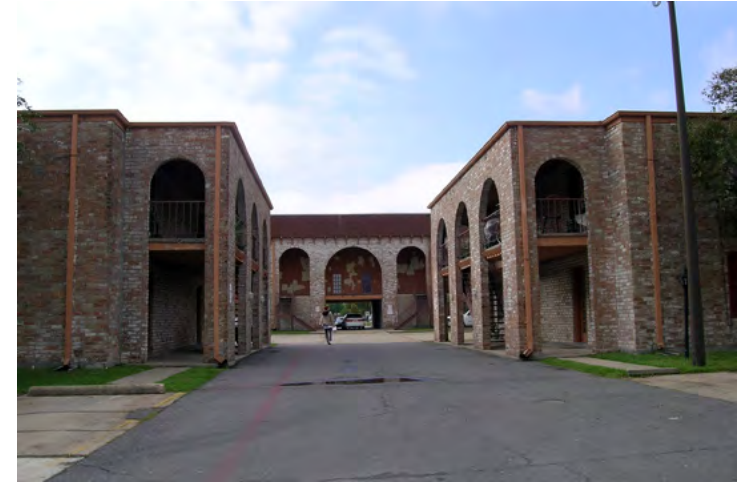
Most apartments in the study area are inward facing like this damaged and partially vacant complex off Whitney Ave.
