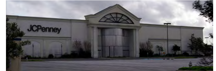
Closed section of the Oakwood Mall
