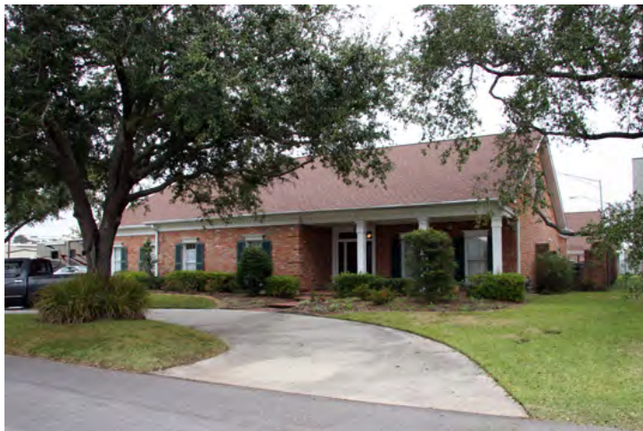
Though historically homes built in the greater New Orleans area were built on stilts, by the 1950s homes were built on slab, a building method unsuitable to a flood-prone area.
