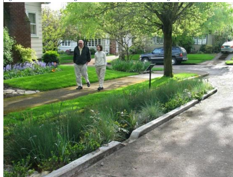
Figure 13: Green Drainage Infrastructure (Portland, Oregon)
