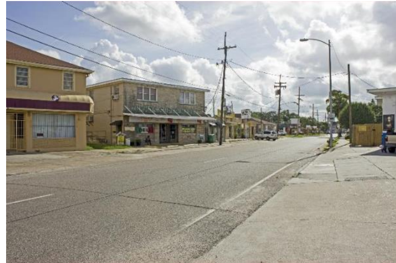
Figure 4: Metairie Road at Severn, Before and After
